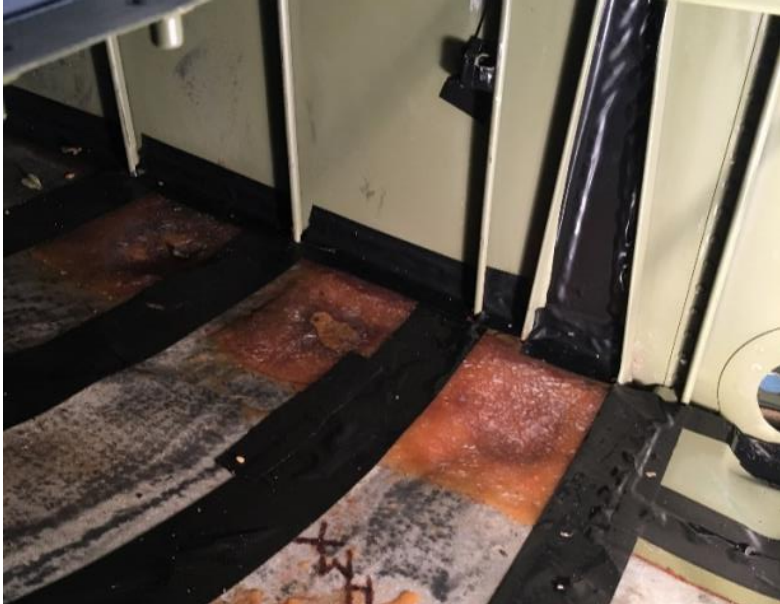
Figure 4.1.4 Fuel Tank Liners and Sealing Tape
