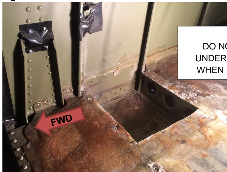
Figure 4.1.7 View of Fuel Tank Liner Removed
