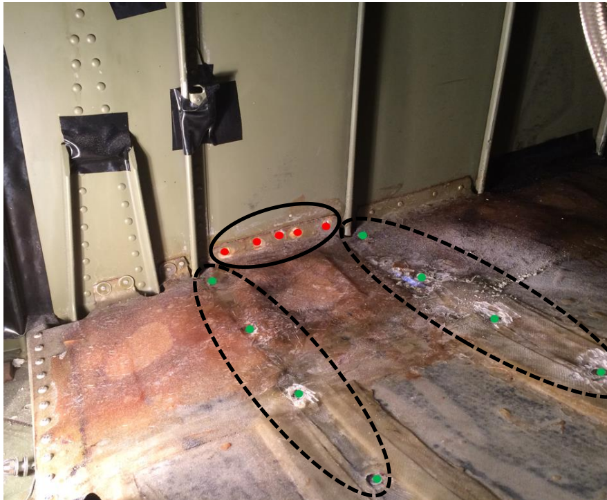
Figure 4.1.5 Rivet Removal for Fuel Tank Liner
