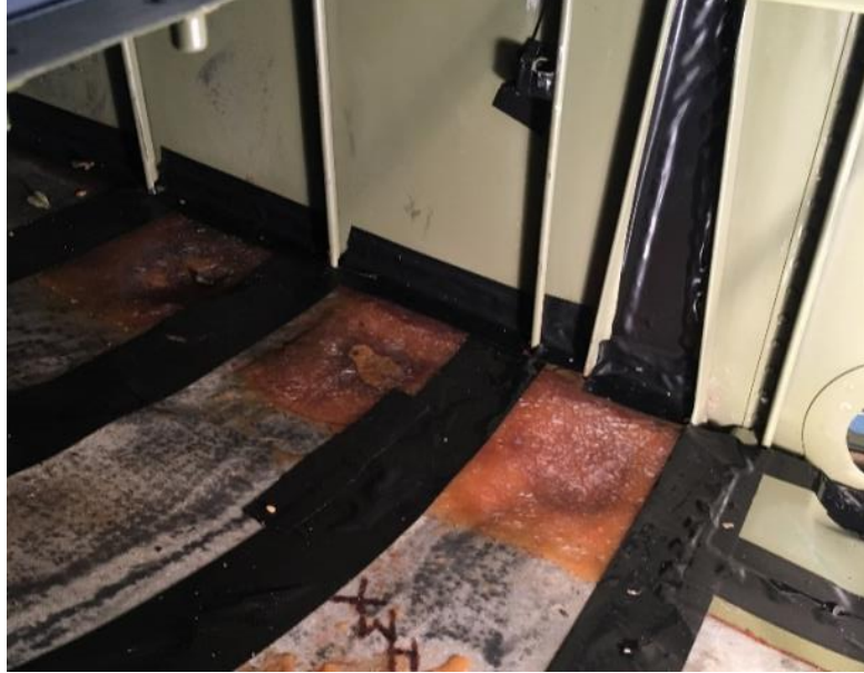
Figure 4.1.4 Fuel Tank Liners and Sealing Tape
