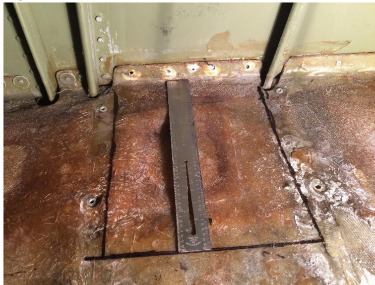
Figure 4.1.6 Liner Access Cut-out at Installation Area
