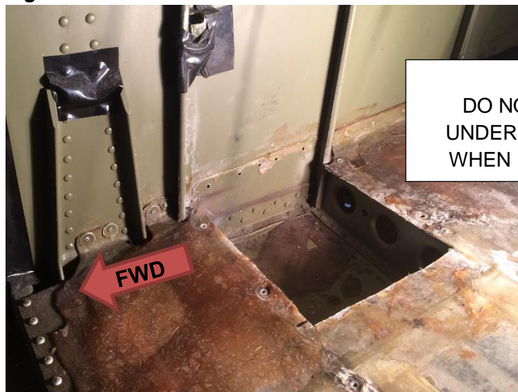
Figure 4.1.7 View of Fuel Tank Liner Removed
